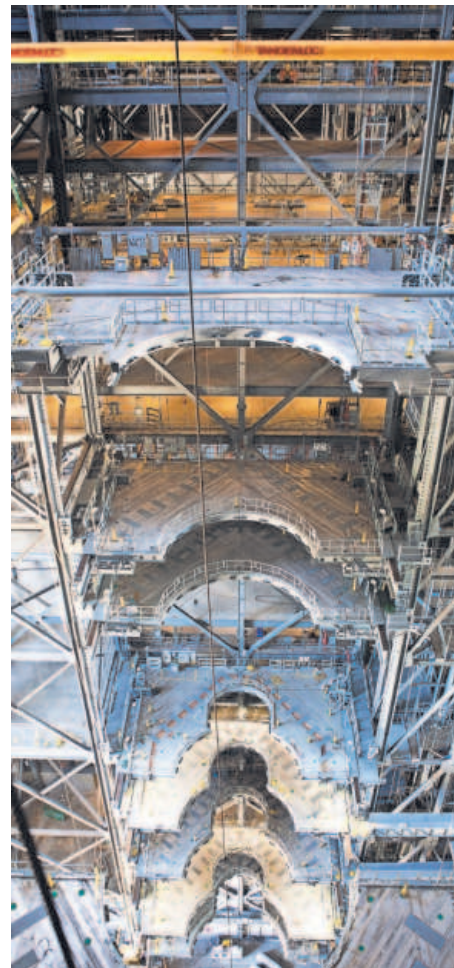
The Vehicle Assembly Building at Kennedy Space Center has new platforms to provide access to the SLS and Orion. DIMITRI GERONDIDAKIS
